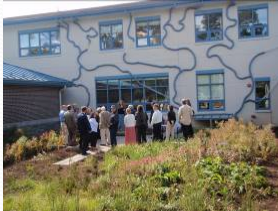
Springside School “Water Wall” and Rain Garden Philadelphia, PA
